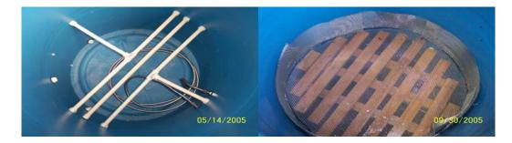
Figure 19: CPVC Pipes Support & Stainless Steel Mesh on Partition
