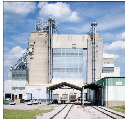
Proper drainage and covering during unloading of product is critical.
